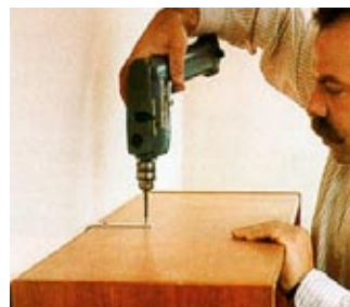
Tall furniture. Bookcases, armoires, and entertainment centers tend to be top-heavy. Secure to wall studs with L-brackets.
